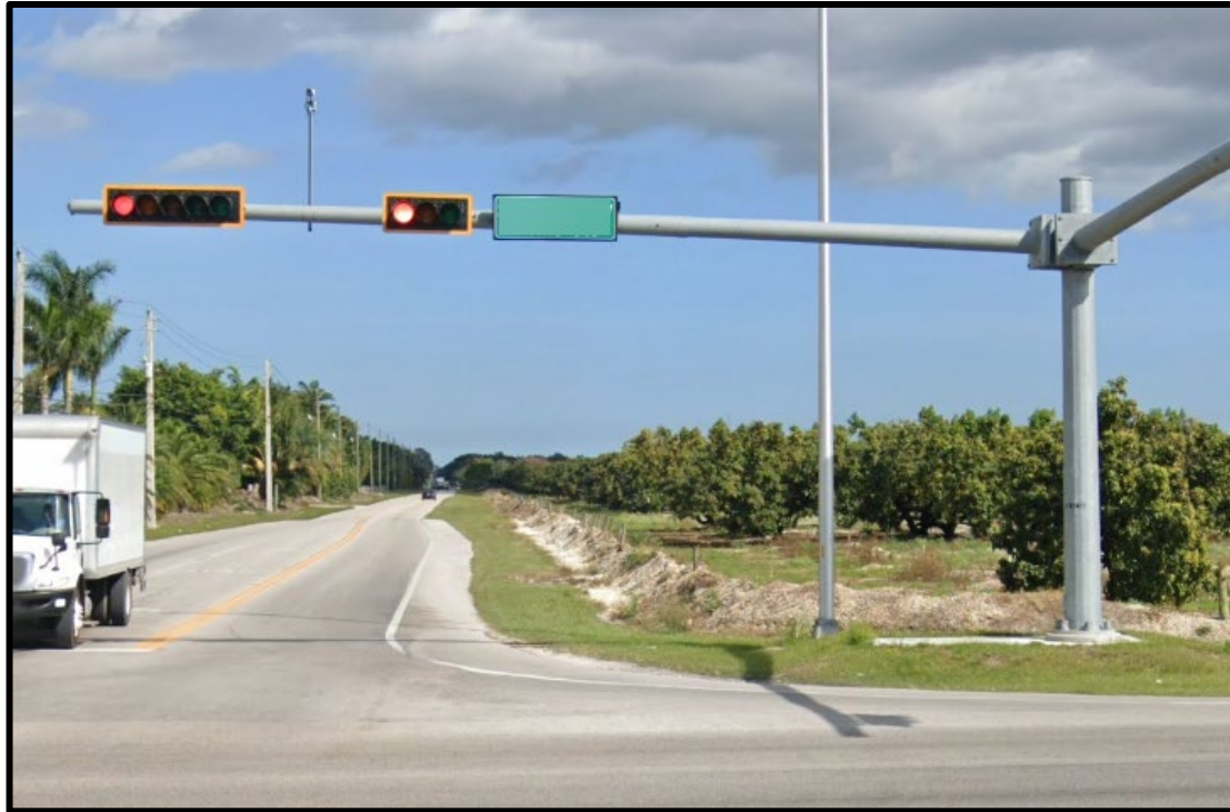
Traffic signal replacement to mast arm system
